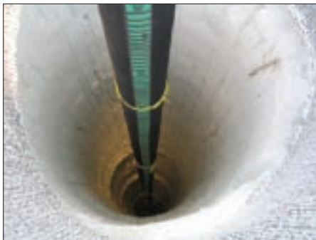
A hose going down into an IceCube hole drilled with the hot-water nozzle
