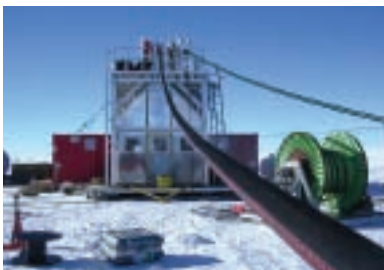
Hosing transports hot water to the drill tower.
